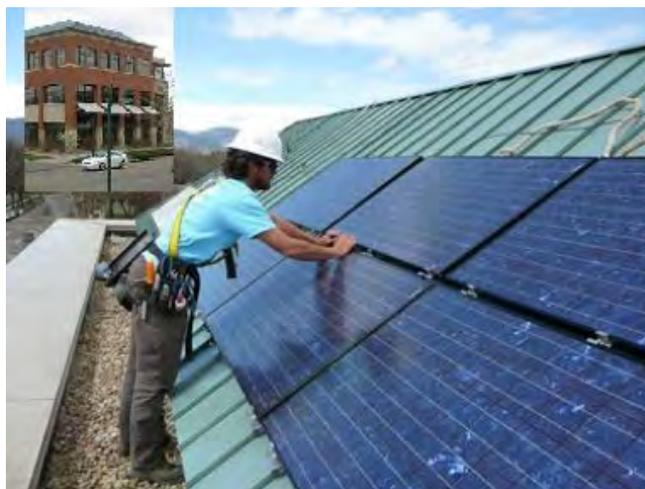
**The city used American Recovery and Reinvestment Act funding to install 6 kilowatts of photovoltaics on the roof of a city office building. Bella Energy installed the system in 2010. Photo Credit: City of Fort Collins**
